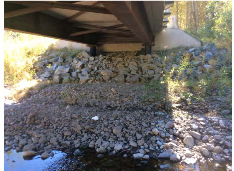
Right Bank Abutment when facing downstream
