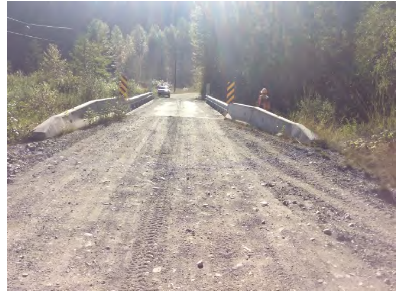
Approach from Left Bank when facing downstream
