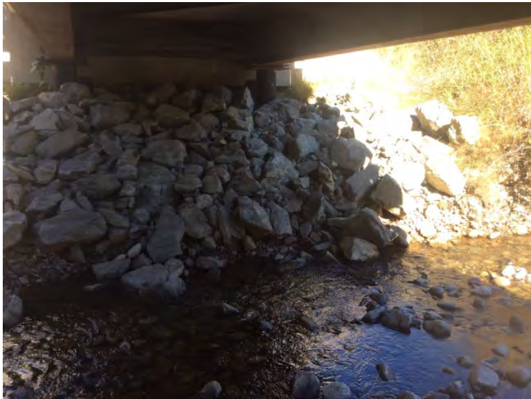
Left Bank Abutment when facing downstream
